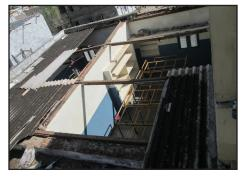
home building had a corrugated roof blown away completely. The doors and windows were damaged as well. But the newer part of the building which is a concrete slab roof was intact. There was great destruction every where in the city. Most of the greenery is gone. I have never seen this much destruction."
